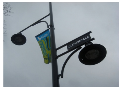
Figure 19. Figure 16. An example of a street light fixture with combined pedestrian-oriented lighting
