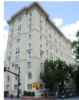
Figure 3. Mt. Vernon Office Building at Charles & Read Streets
